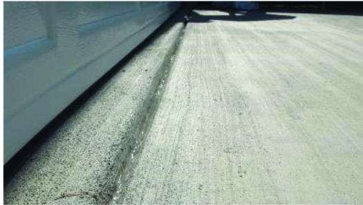
(c) Garage door, driveway, and expansion joint
